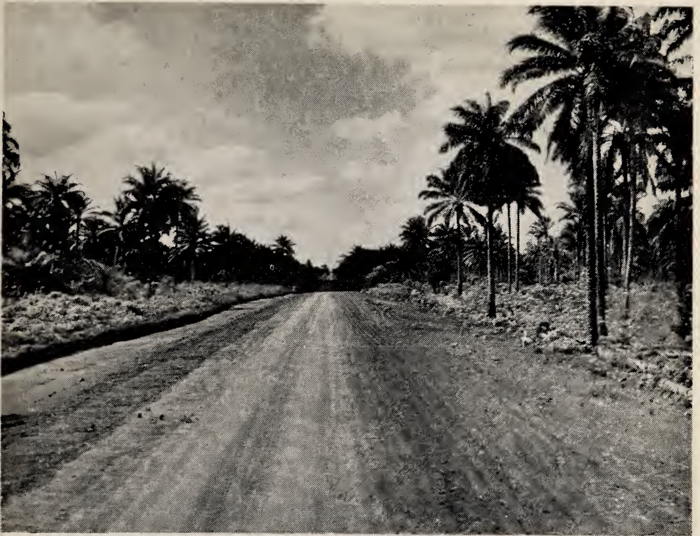
A TRUNK ROAD CONSTRUCTED UNDER THE DEVELOPMENT PLAN
